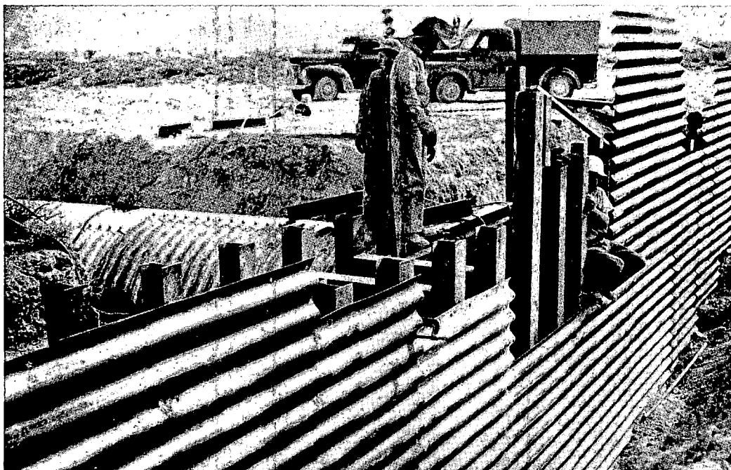
Fig. 4—Erecting steel Multi-Plate ramp entrance.
